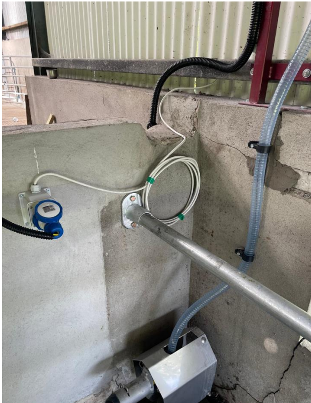
Fig 11. Installation of wiring and permanent water source for scraper units
