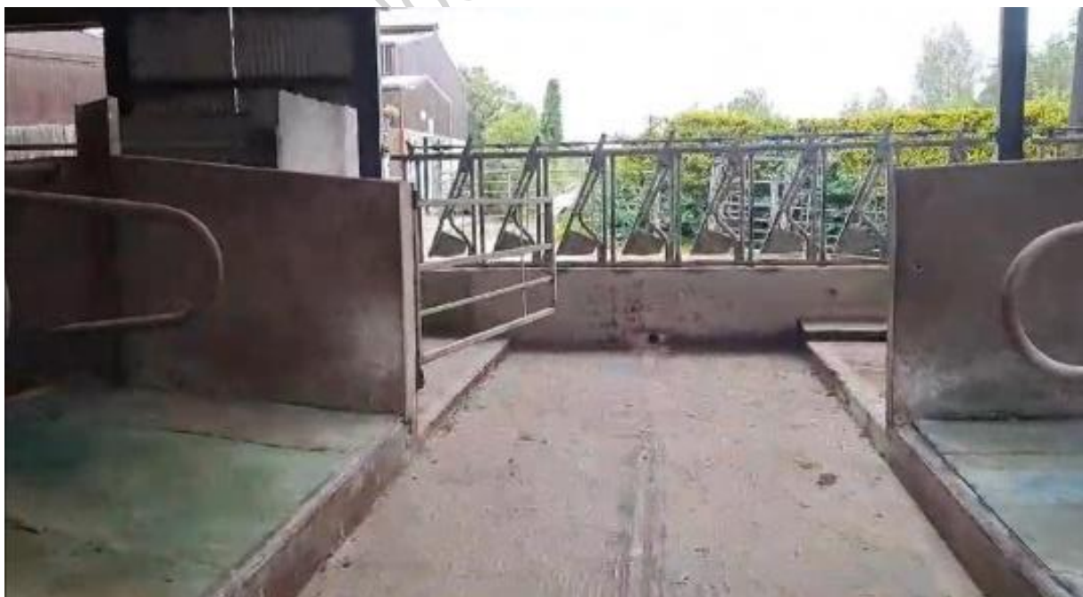
Fig 1. Existing passageway with steps to either side. These had to be removed and entirely new concrete passageways laid
