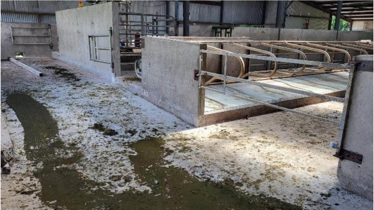
Fig 3. New passageway demonstrating the change in height and significant changes needed to accommodate the scraper.
