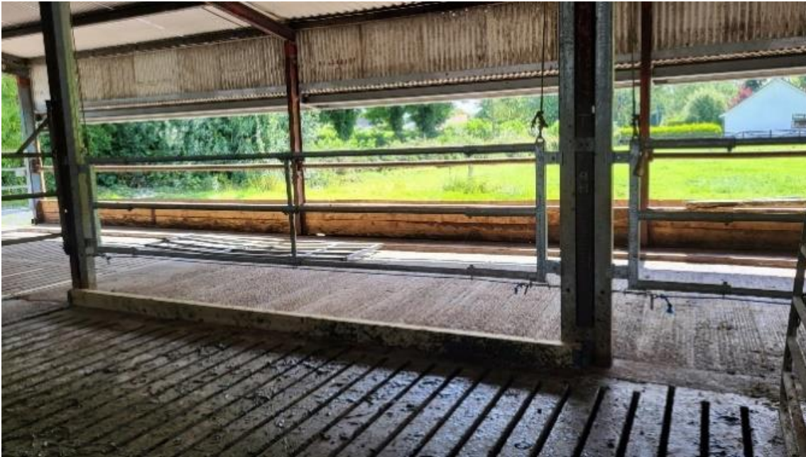
Fig 5. Passageway separated via installed barrier bolted to plates welded into place to reduce the size of the passageway.
