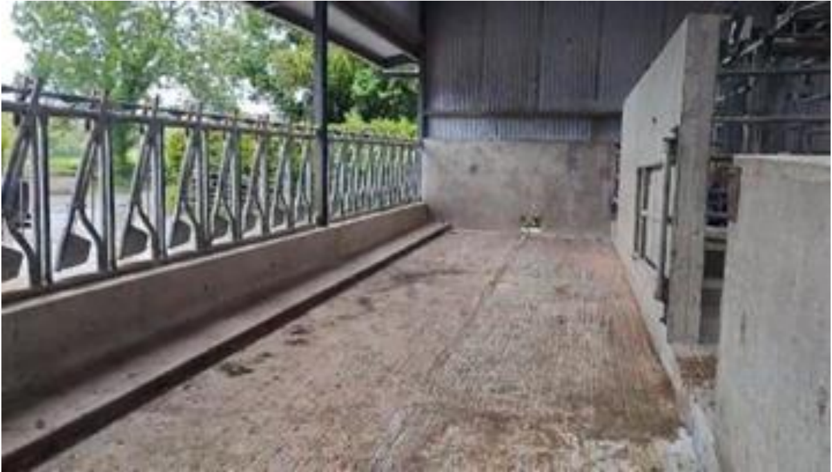
Fig 2. New passageway laid complete with step to guide scraper (near feed barrier)
