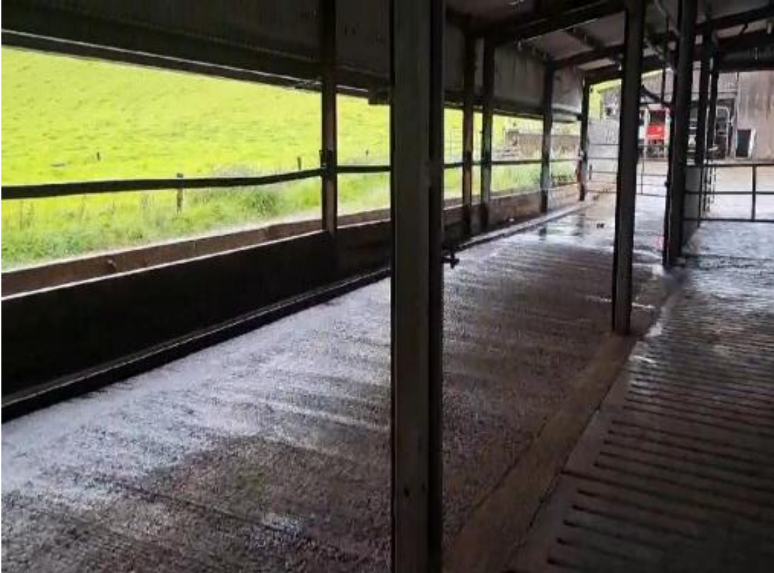
Fig 4. Passageway of over 5m, too wide for robotic scraper
