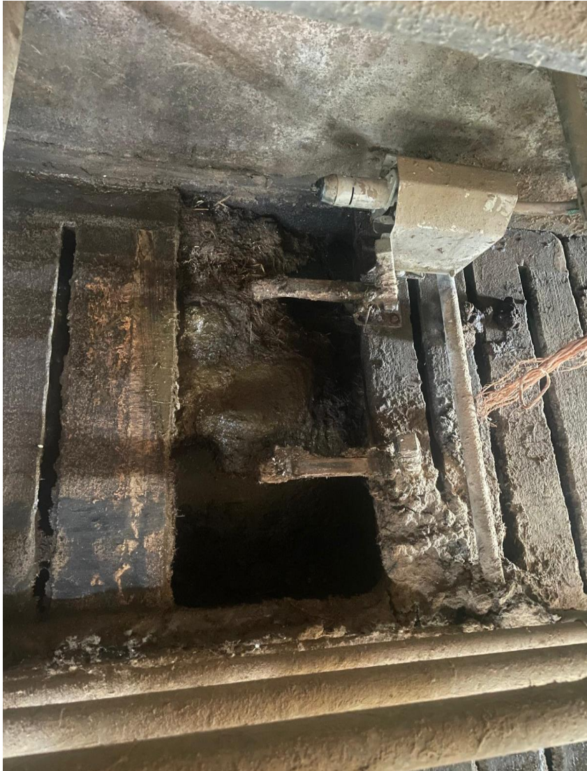
Fig 8. Specifically build sump for Lely Discovery Collector to deposit collected manure.
