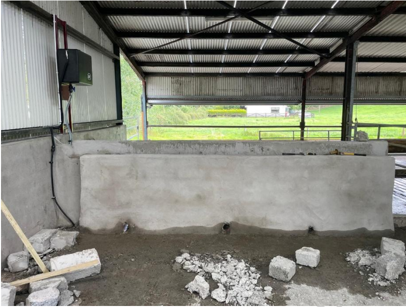
Fig 9. Structural work required to install Lely Discovery scraper
